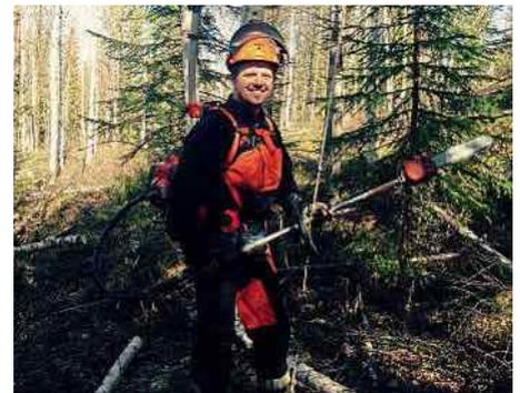
Clearing the boundary with a special saw – a hybrid between a brush cutter and a pole saw
