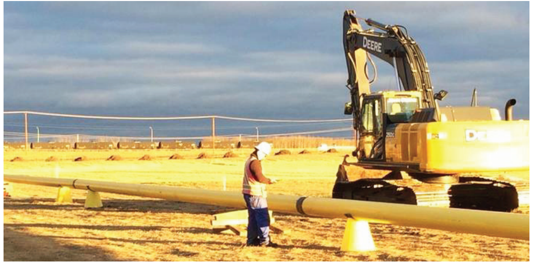
Lance Fugate of Enmapp inspects pipeline construction using the Arrow 100, TerraGo Edge on iPad in Canada.
