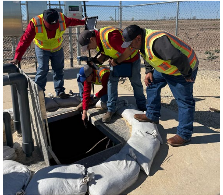
The EPWWS GIS team use the Skadi Smart Handle, Skadi 300 GNSS receiver, and ArcGIS Field Maps to map inside a pump station vault. The technology combination allows the team to "point-and-shoot" into the vault.
